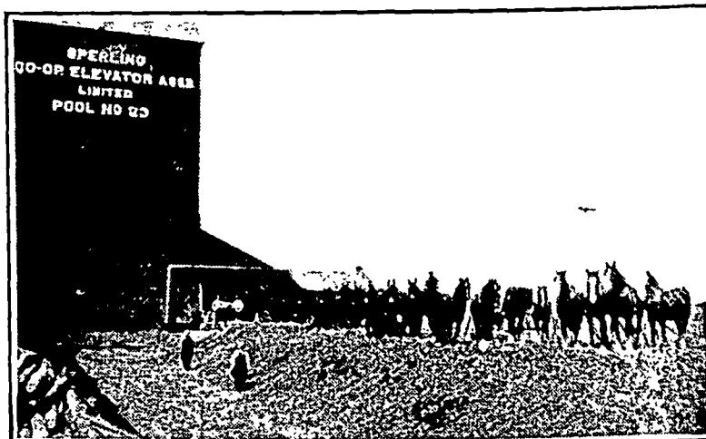
"The gang goes to it at Sperlino Elevator. The excellent runway is being put in to save horseflesh and the damage to wooden runways from tractor wheels."
